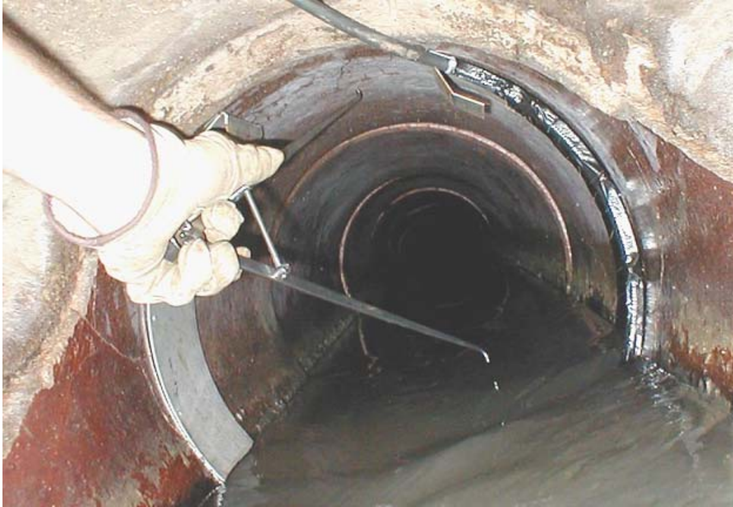
Field Check of Level after Installment
